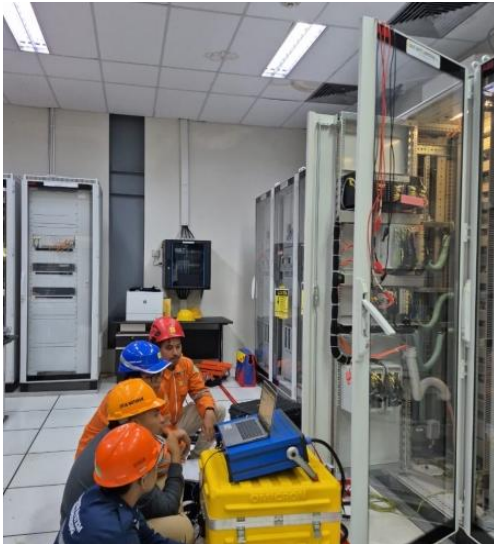
Gambar 5. Proses Pengujian Distance Relay di GI 150 kV Sengkol
