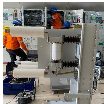
Gambar 3. PMT SN 7 GI Paniki
